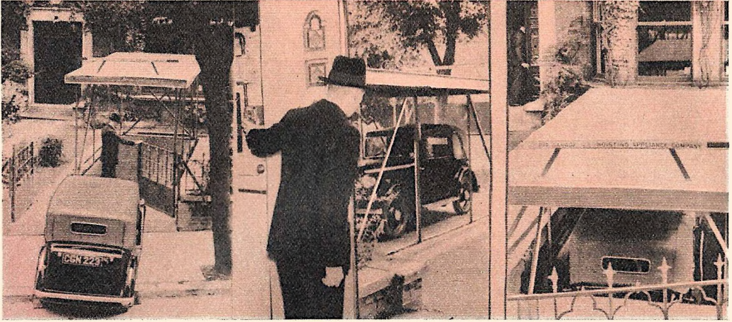
Restricted by law from building a regular garage on his lawn, a London suburbanite solved the problem by installing an electrically driven elevator garage under the lawn. Controlled by switch (center photo), the elevator quickly rises or descends.
