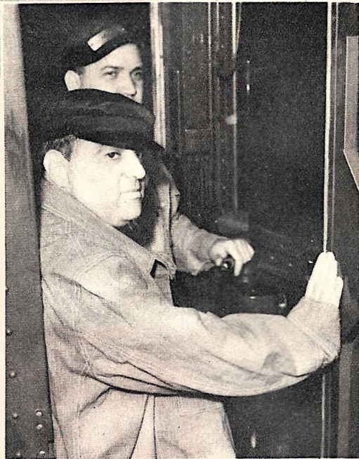
Left—New York's mayor, Fiorello La Guardia, in the control cab of the train that opened the new link of the Independent Subway connecting Queens and downtown Brooklyn. Top—A quick-accelerating, short-stopping train of the Independent Subway pulls into the Hoyt Street station. Subway stations are brightly illuminated and well maintained.
